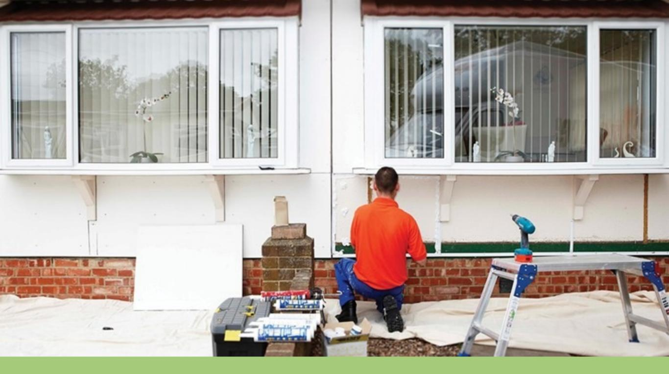
Insulation panels are fitted to the outside walls of your park home by specially trained technicians. Joints are sealed with silicon and then covered with scrim tape and plaster, before a smart outer layer of stippled paint is applied.
